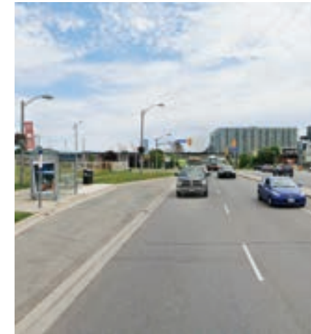
4 Existing condition along Wilson Avenue
