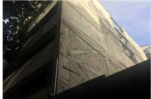
Fig. 6: Confined masonry frame with St. Andrew's cross bracing (SOM).
