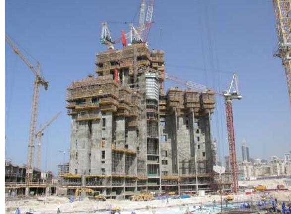
Figure 23 – Self-Climbing Formwork System
